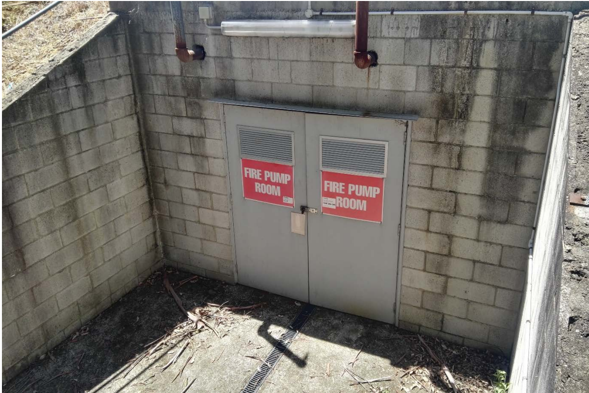
Photograph 10: Fire Pump Room entrance built in to slope
