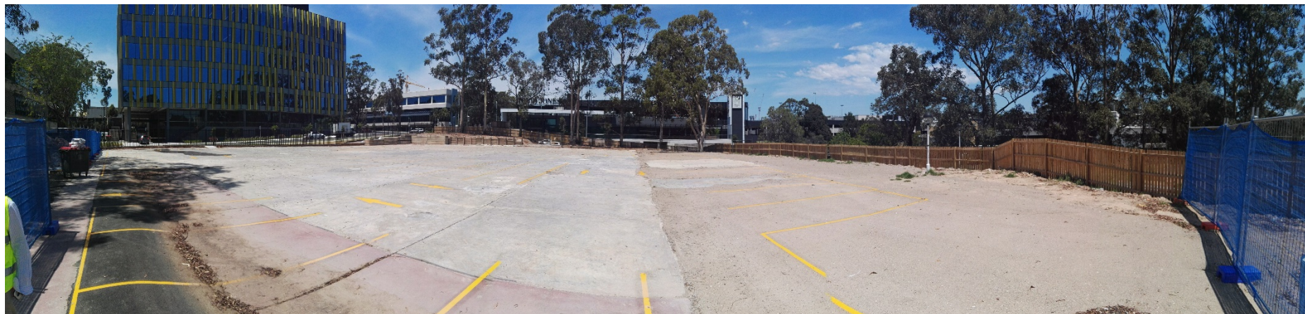
Photograph 3: Floor slab of the recently demolished building.
