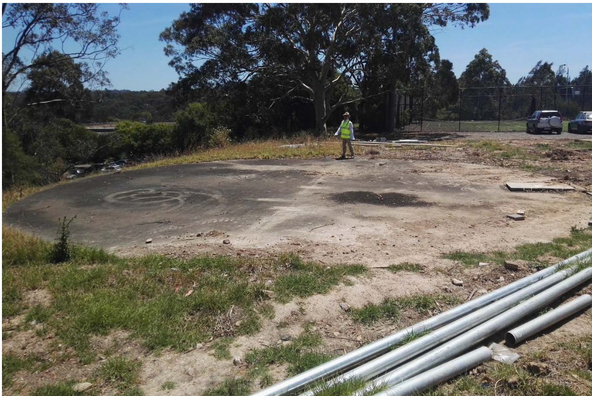
Photograph 11: Large diameter concrete slab above the Fire Pump Room.
