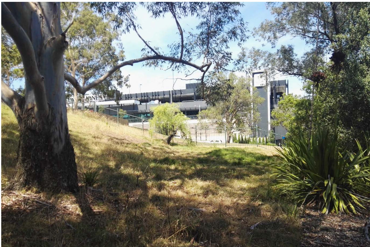
Photograph 5: Benching of site slopes
